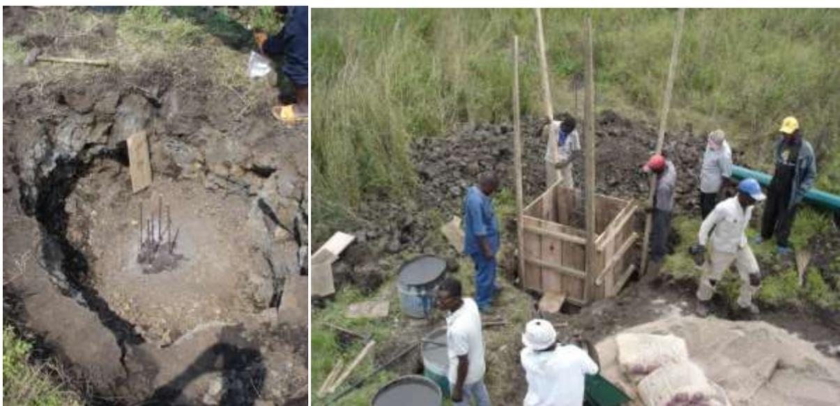
**Figure 22: Anchoring the monument to the base rock at Rusayo station (left) and building of the concrete base (right).**
